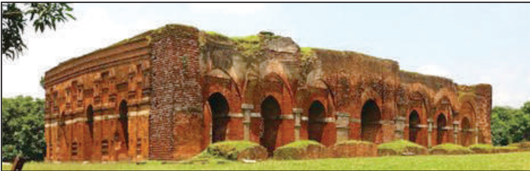
Darasbari Mosque of Chapainawabganj
