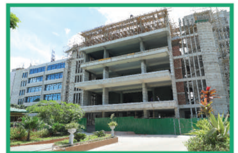
Ongoing Development Activities of BUP
